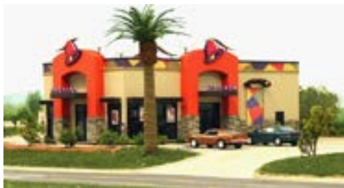
#TB-003 New Taco Bell Restaurant
